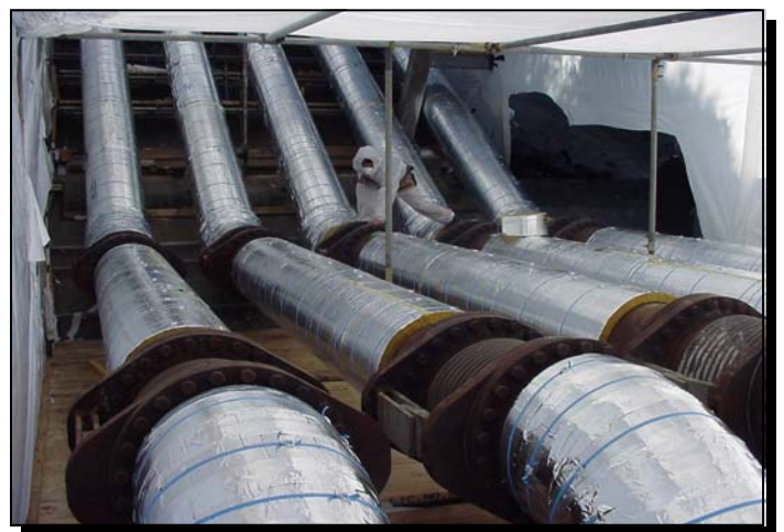
Glass wool faced with aluminium foil to act as vapour barrier around pipes.
